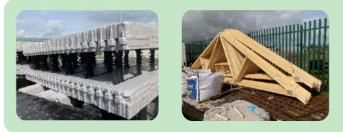
Figure 24: ICF module & roof truss
