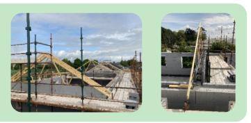
Figure 26: External ICF wall, part wall, and roof truss
